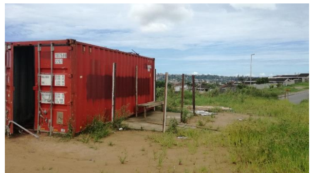
Figure 23 | Abandoned container on erf D
