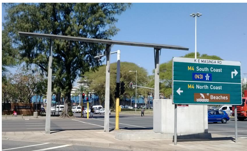
Figure 1: Solar Powered Traffic Signal System
